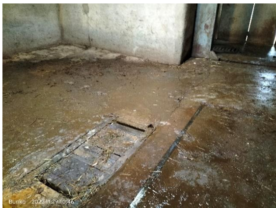
Fig. 26 – Gully cover and concrete floor
