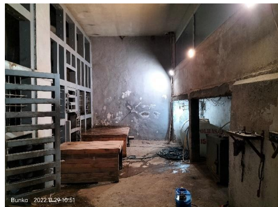
Fig. 17 – Staff corridor and flood lamps
