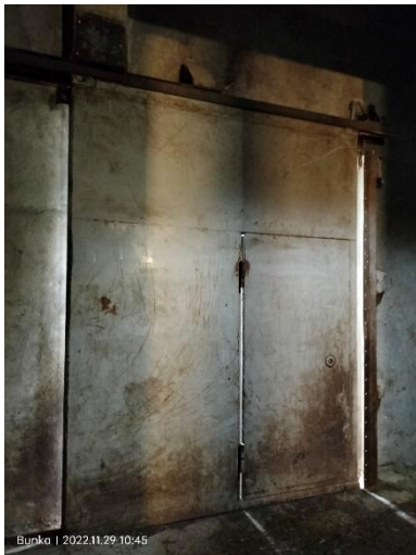
Fig. 20 – Steel gate to outside yard
