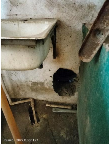
Fig. 22 – Fan heater outlet into staff corridor
